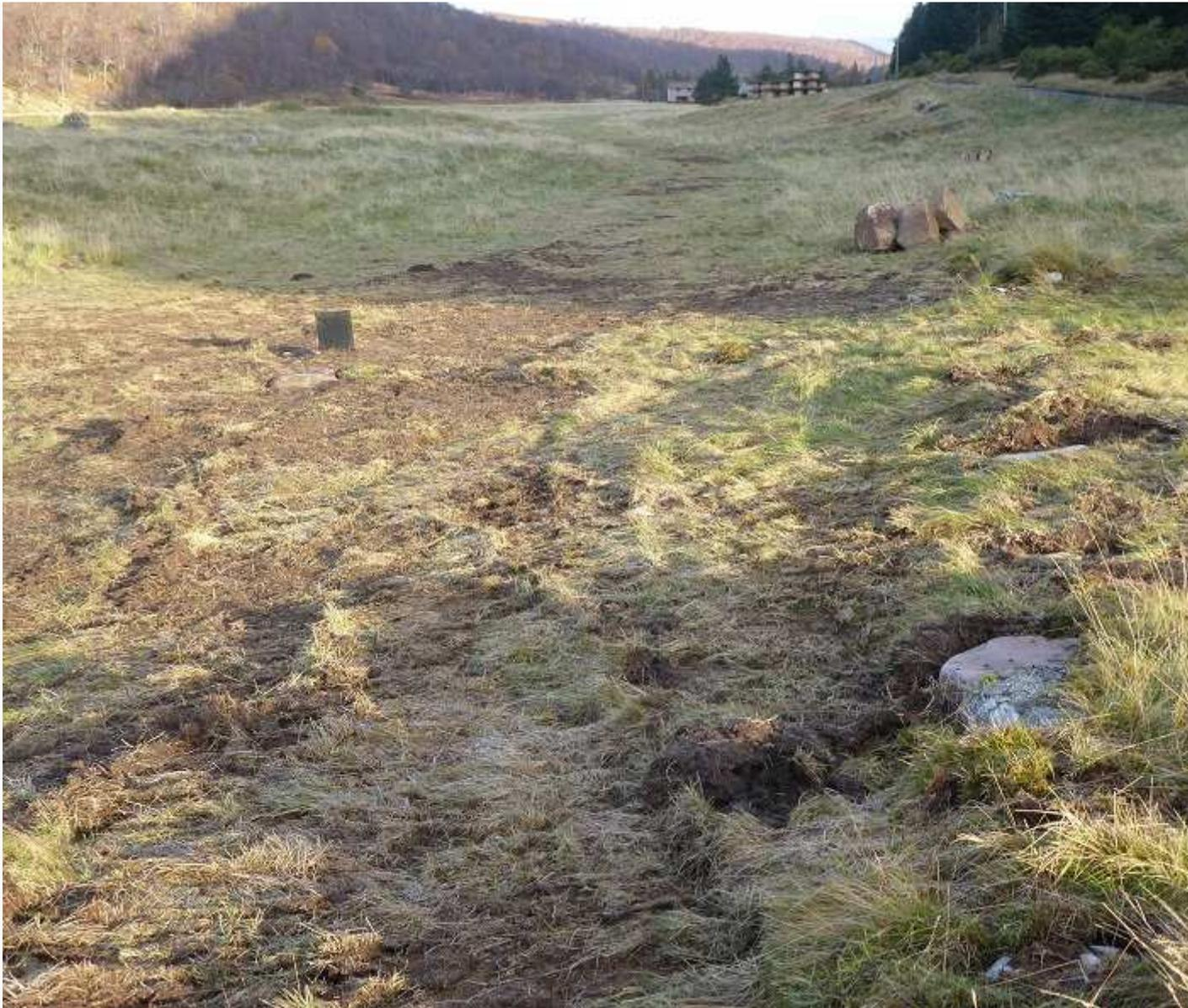
You can however see some evidence that a mole plough has been used. In places boulders have been excavated to allow the passage of the plough and cable.
